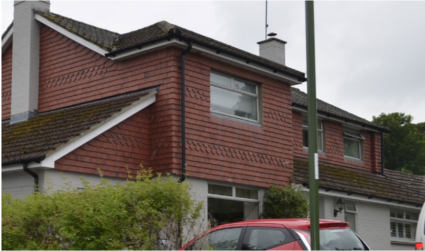
WHITE WEATHERBOARD AND HUNG TILE ON UPPER FLOOR
