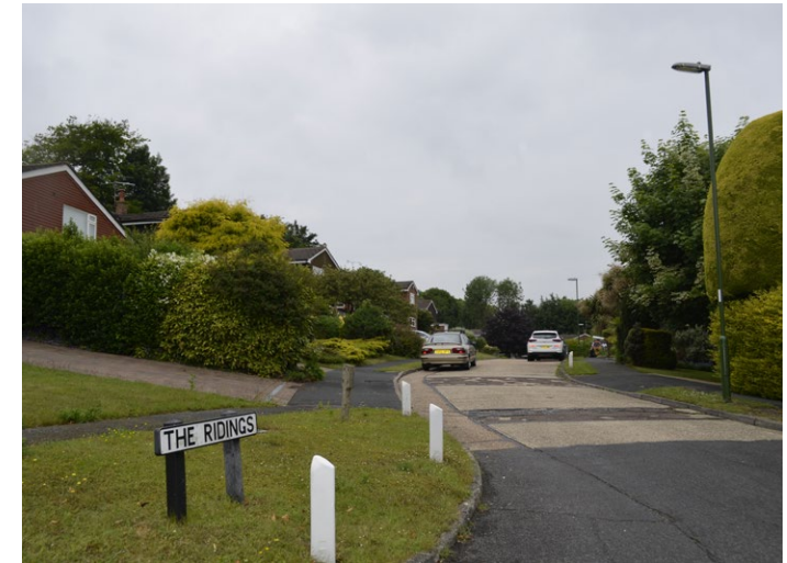
Sloped access to houses at the Ridings
