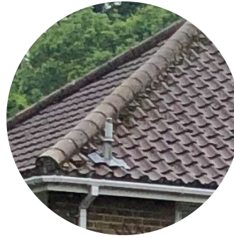
PANTILES ON ROOF
