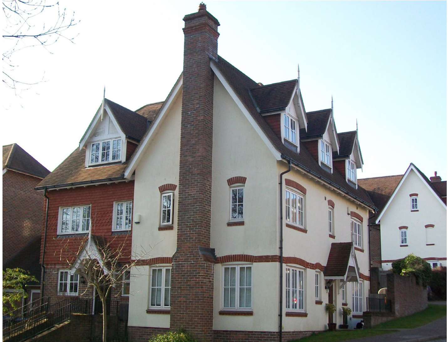
Linked dwellings at the corner with articulation of the built form and windows opening onto both frontages
