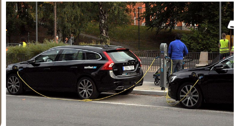
Inset parking with electric vehicle charging points.
