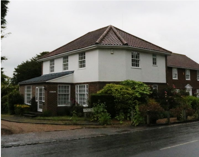
Example of effective corner treatment in Bramber
